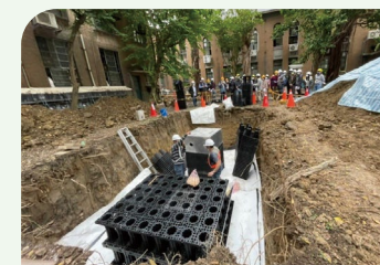
Laying Water Harvesting Modules to improve drainage in the courtyard.
